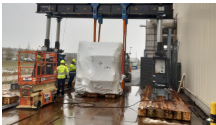
Manipulating a 54T press at a chemical plant in Ghent
