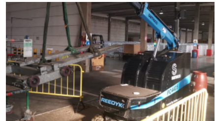
Installing equipment with our 3T Reedyk EX crane at Lanxess Antwerp
