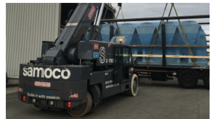
Placing a Chiller on the roof at Fujifilm
